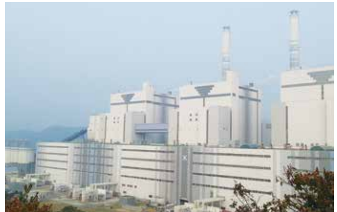
Far view – Yeongheung Thermal Power Plant.
