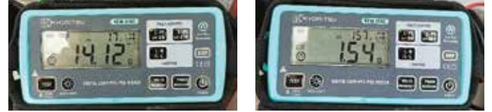
(c) Earth loop impedance test -- Earthing rods without connection to foundation steel re-inforcing bars
